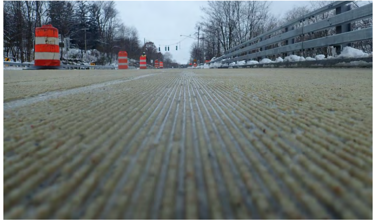
Grinding with Slurry Removal (557.60010004)
