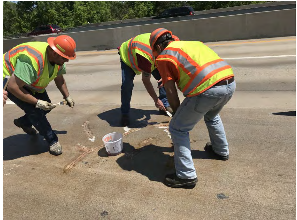
Applying HMWM to treat crack on the overlay.
