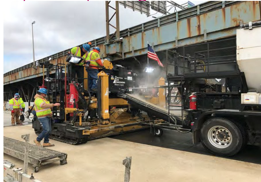
Slip-form paving machine
