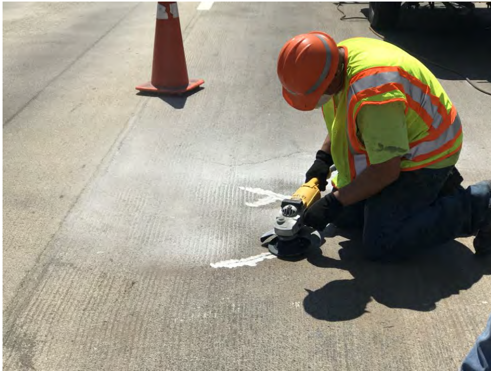
Applying HMWM to treat crack on the overlay.
