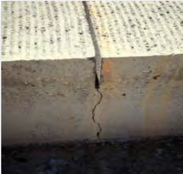
Conventional Sawcut \frac{1}{4} to \frac{1}{3} of thickness
