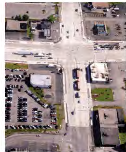
An intersection reconstructed with concrete.
