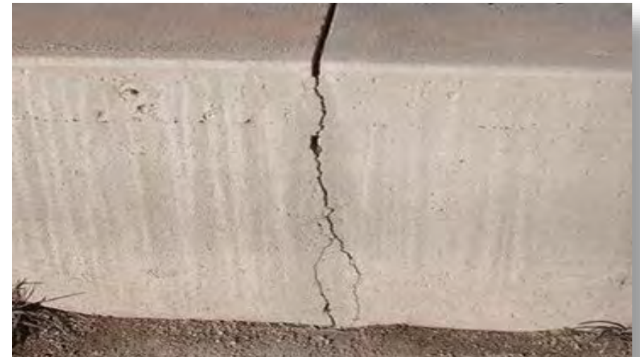
Early Entry Sawcut ~1 inch
