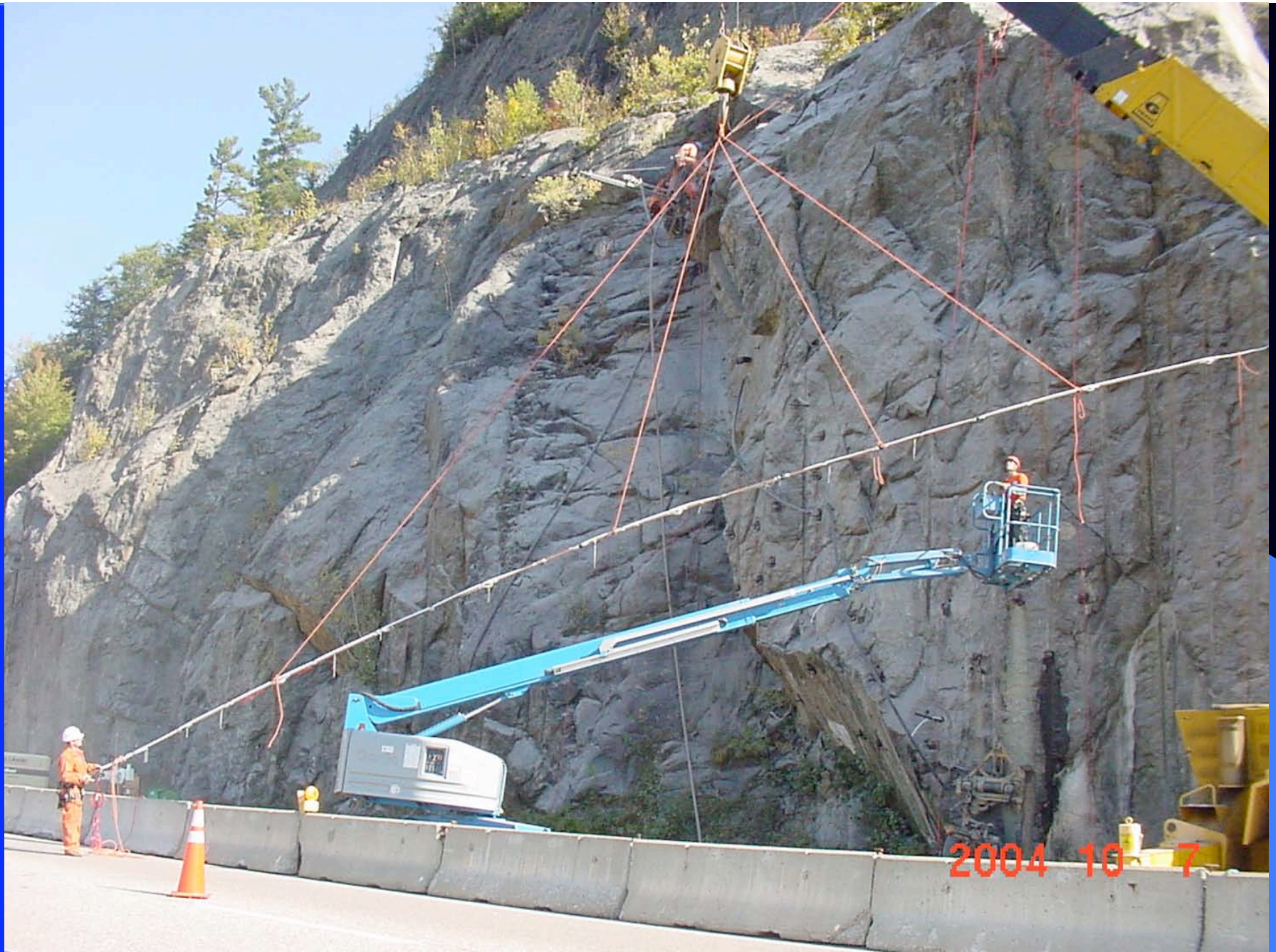
Installing Rock Tendons
