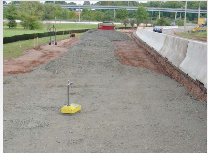
Southington, CT site
