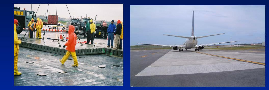
2 test sections – 16 in. & 12 in. prestressed panels – 25 long by 12.5 ft wide
