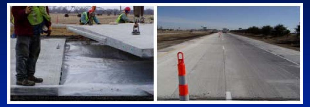
Replaced two pavement lanes and added integral shoulders on both sides
