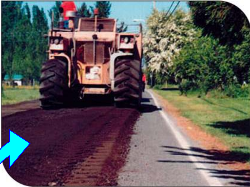
1. Pulverize the old road or existing subgrade
