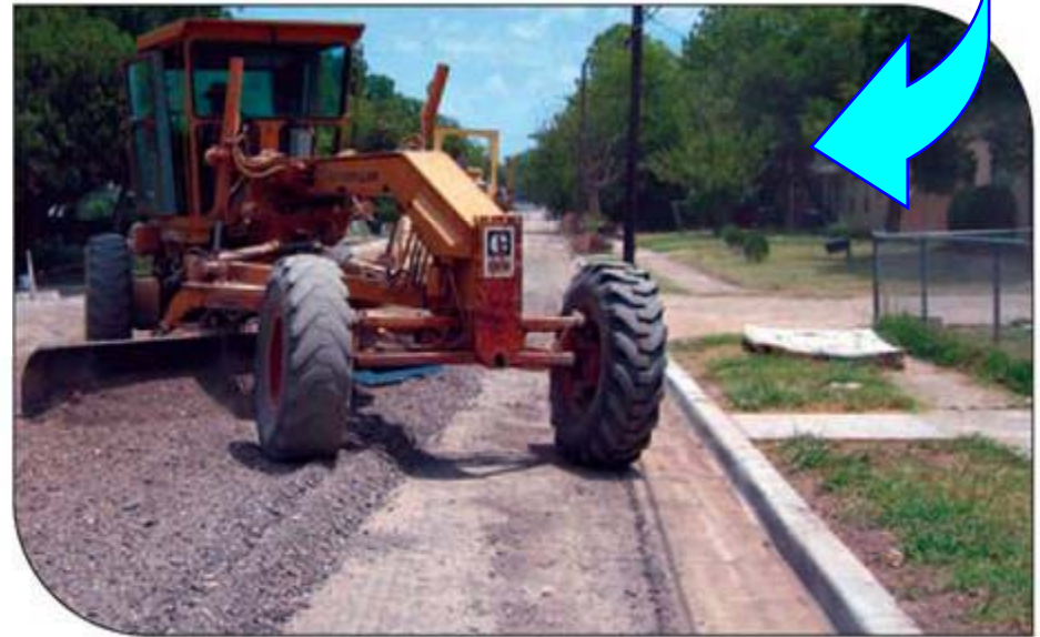
2. Initial shaping and grading
