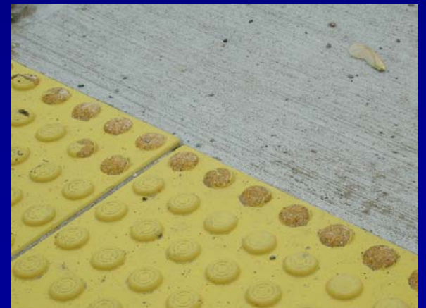
Dome loss/scraping
