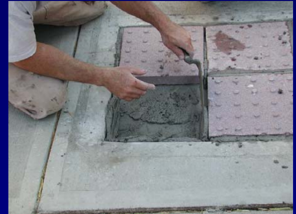
Granite pavers mortared
