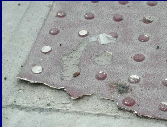
Delamination
