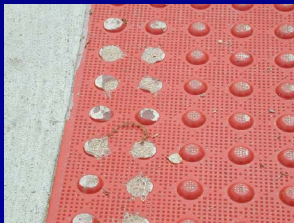
Dome loss/scraping
