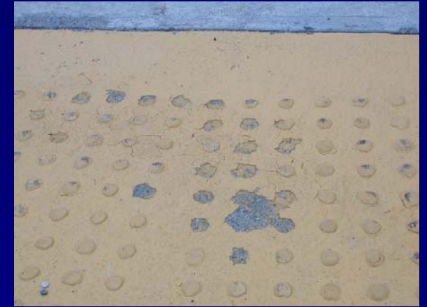
Dome loss/base loses adhesion
