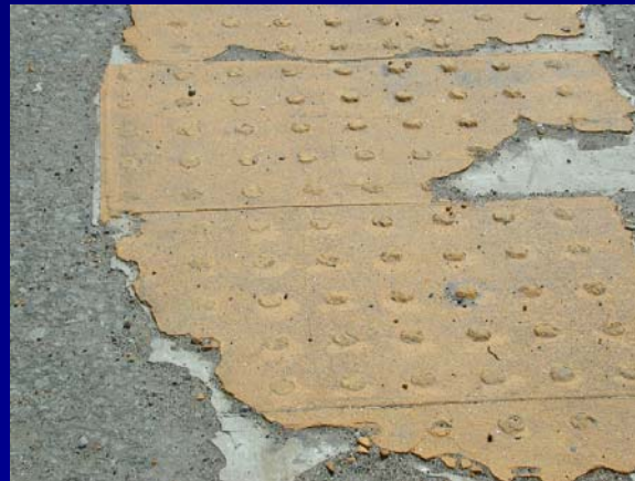
Delamination/dome loss
