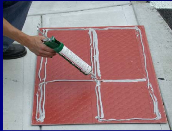
Adhesive under panel
