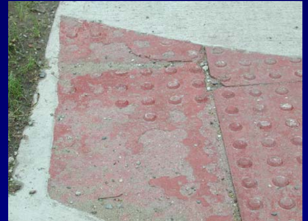
Spalling/domes crushed
