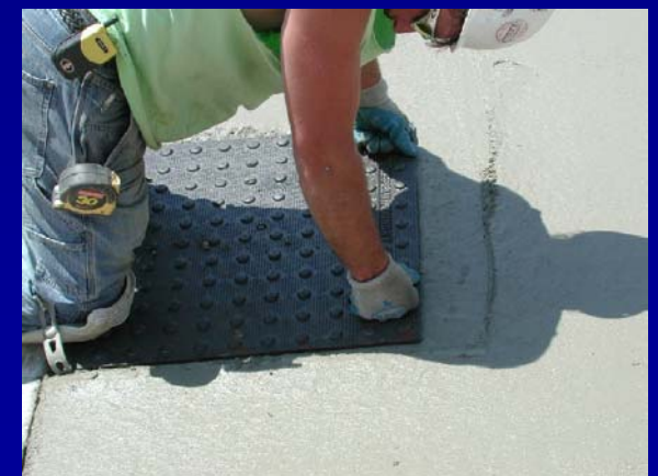
Cast iron cast in place
