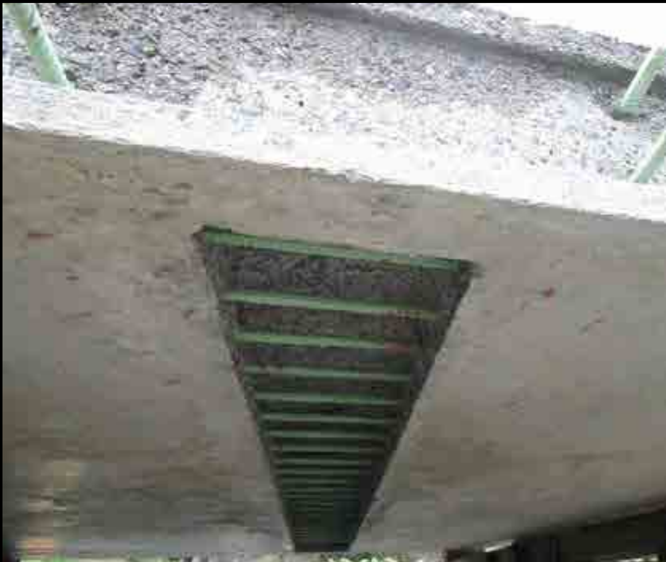
Deck-to-Girder Connection
