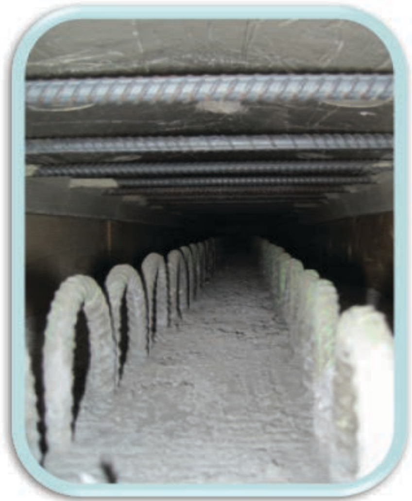
Concrete Girder Connection
