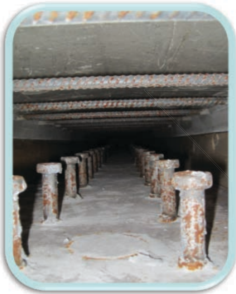
Steel Girder Connection
