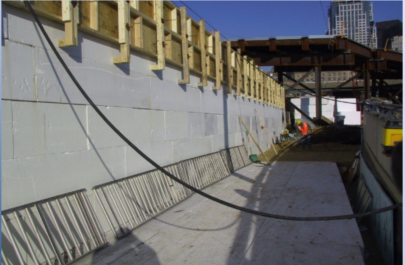
Temp Ramp KK - Advancing Block Placement
