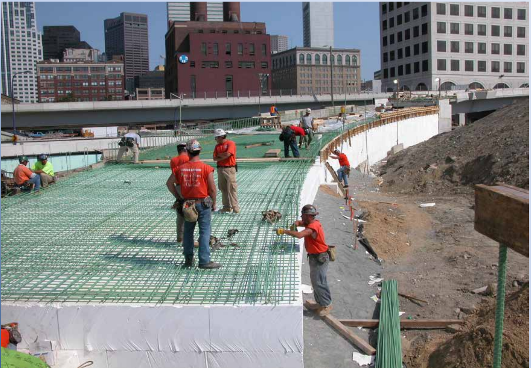
Curved Ramp F under Construction
