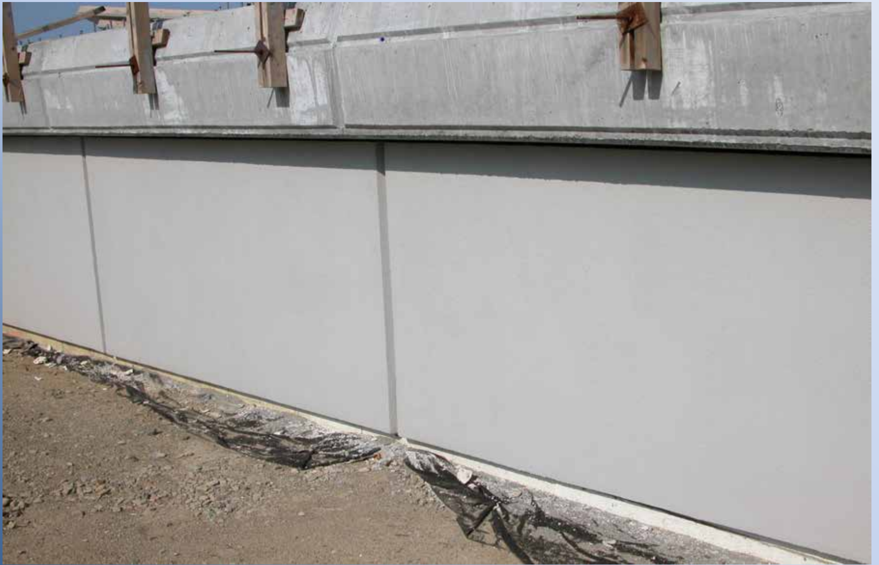
Finished EIFS – CA/T - Ramp X
