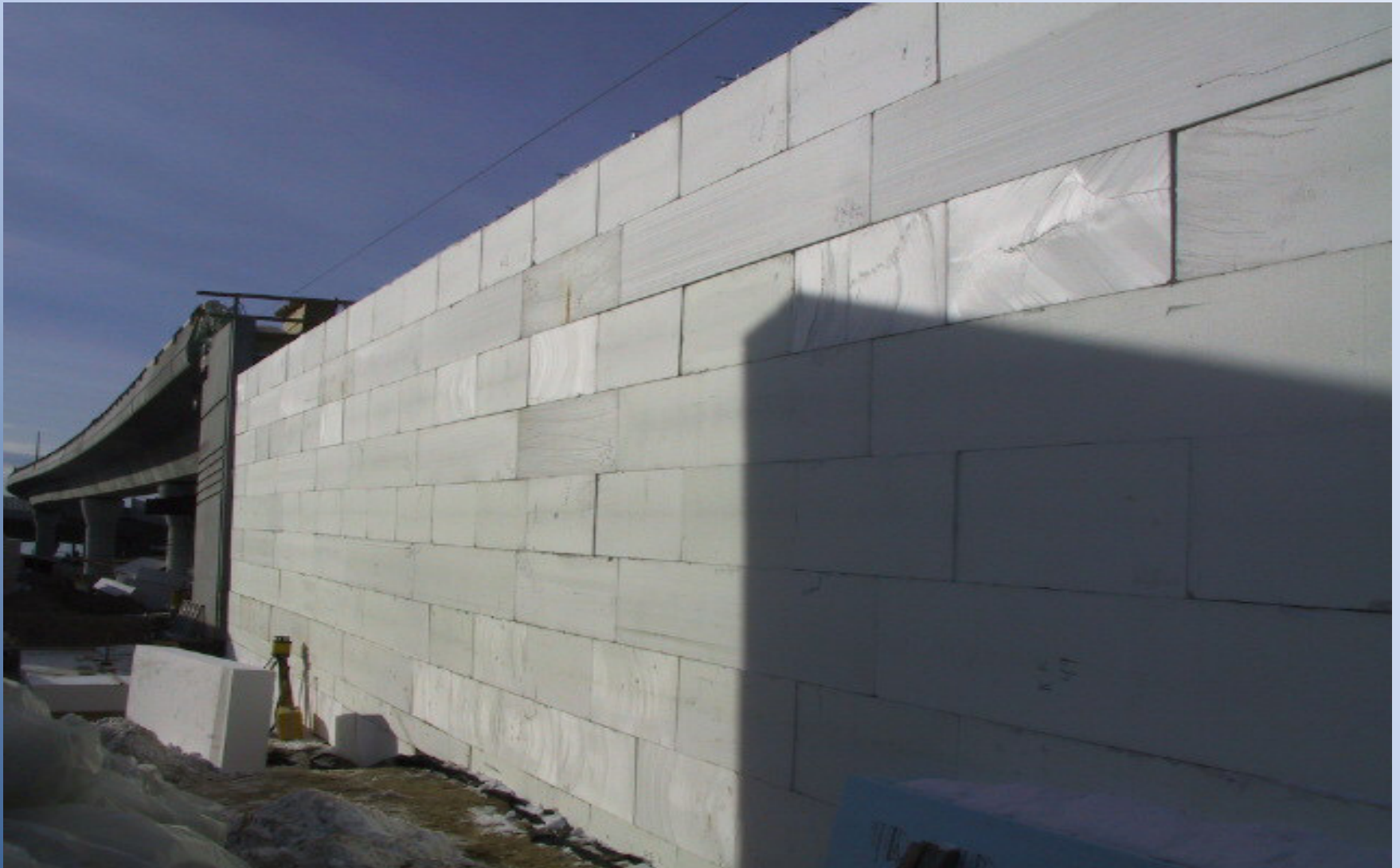
Permanent Ramp KK - Blocks Assembled East Side
