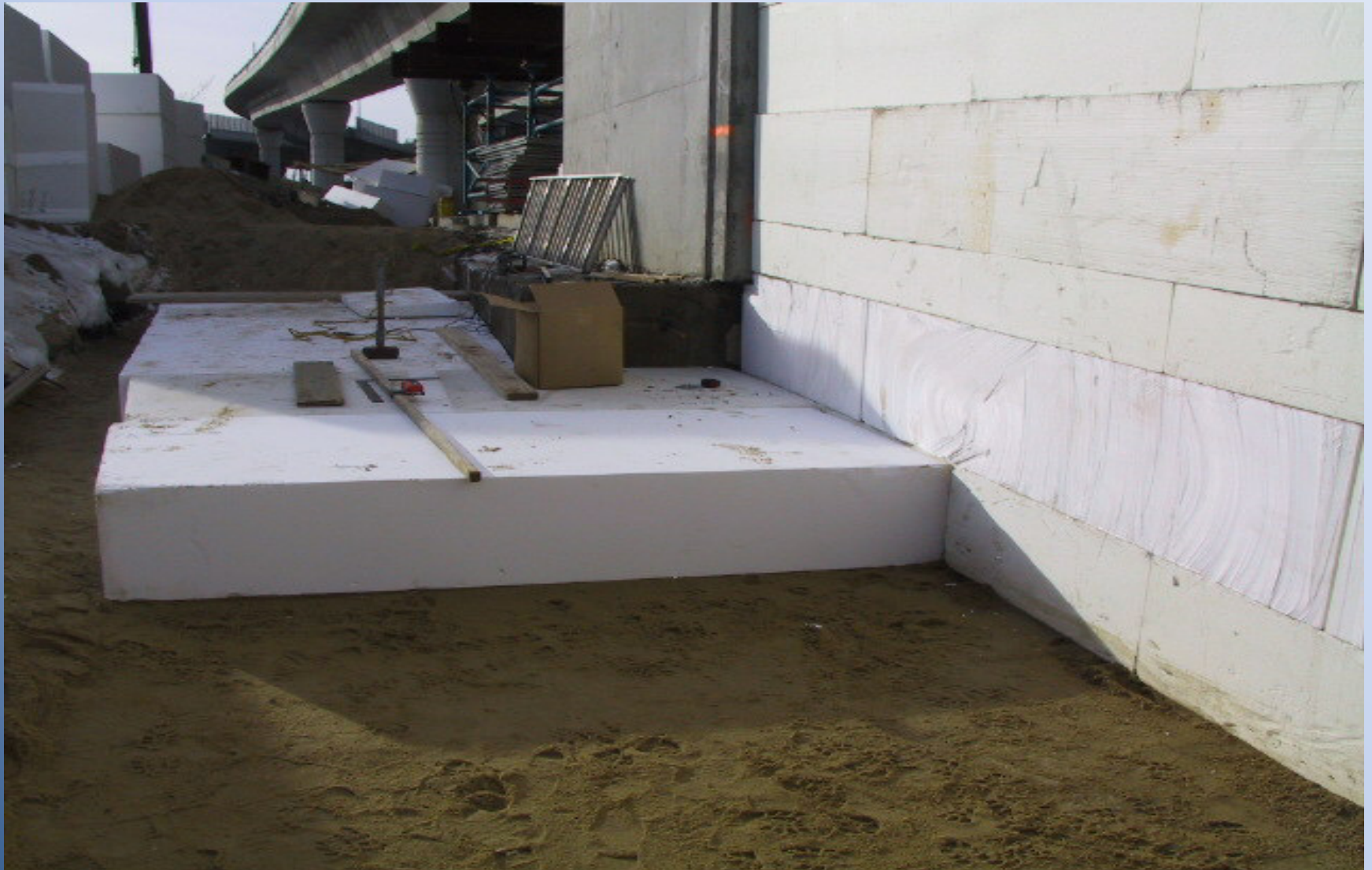
Temporary Ramp KK - Early Blocks Placed
