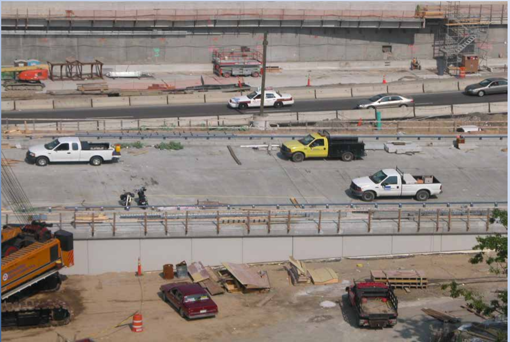
Finished EIFS – CA/T - Ramp X
