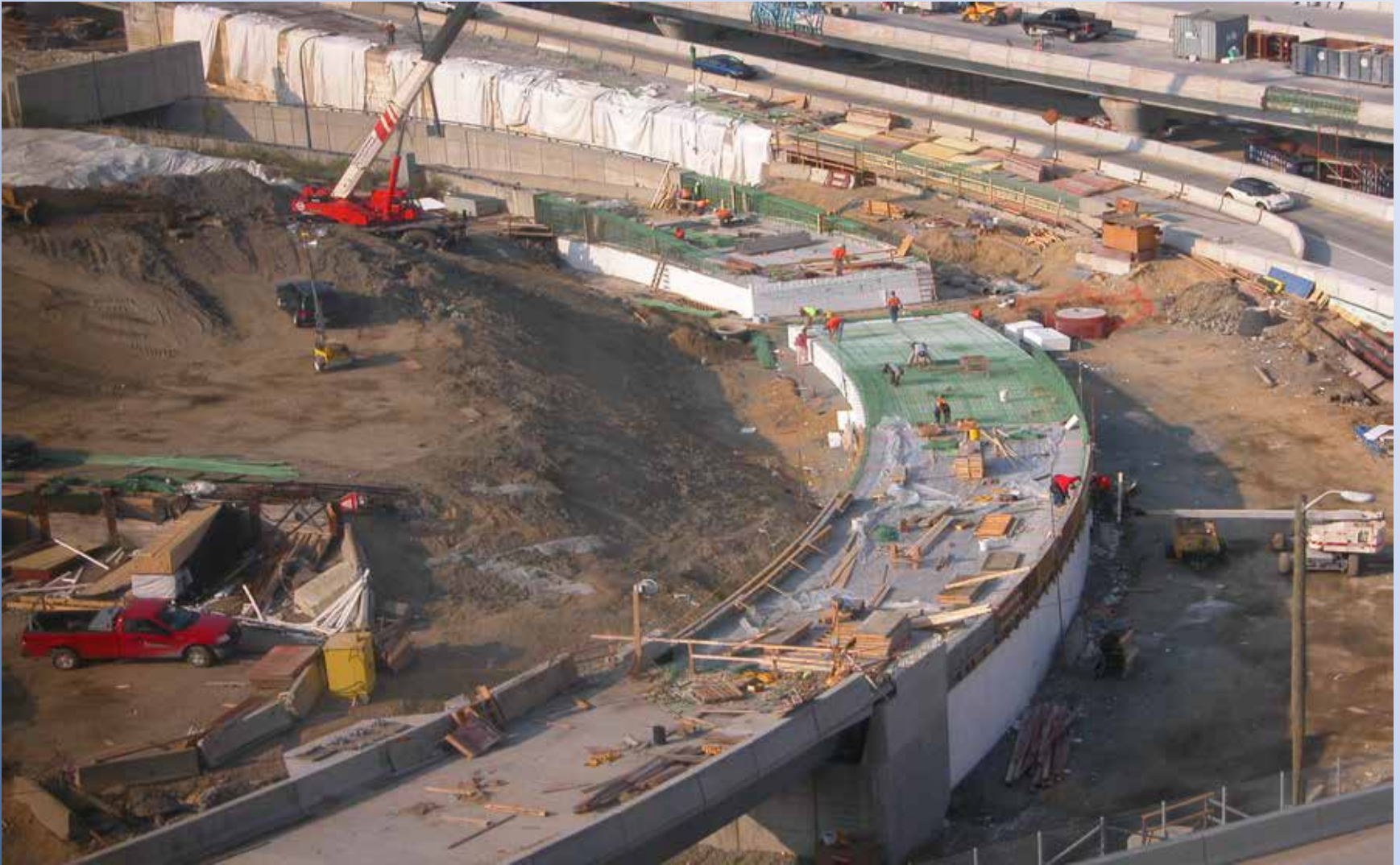
Temporary Ramp KK Demo Complete Curved Ramp F under Construction
