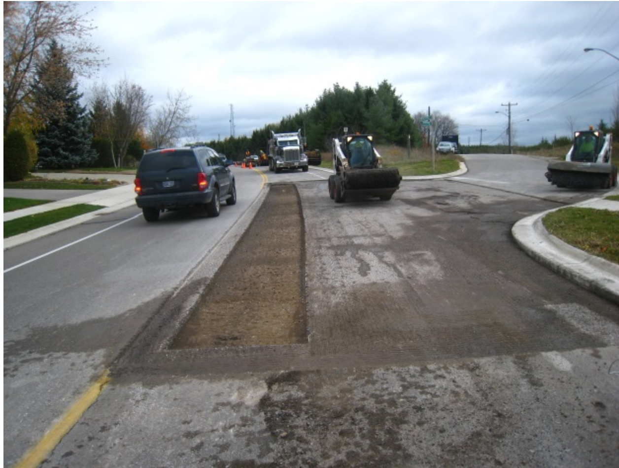
Repairs of new binder course that incorporated high amount of RAS
