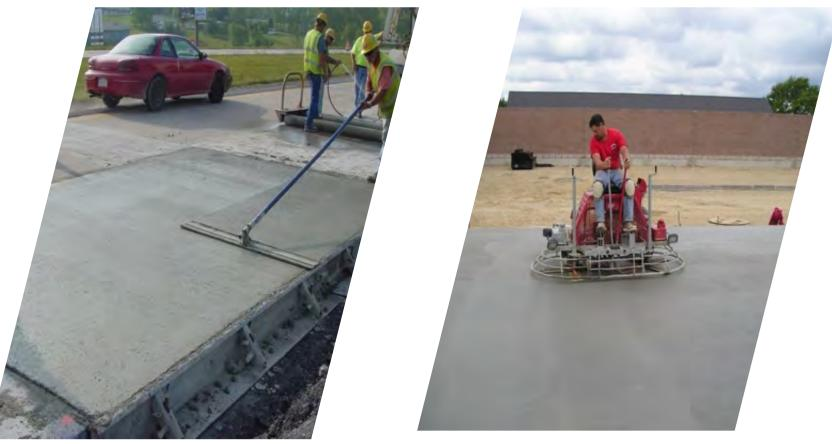
FRC can be finished with similar tools as used for unreinforced concrete.
