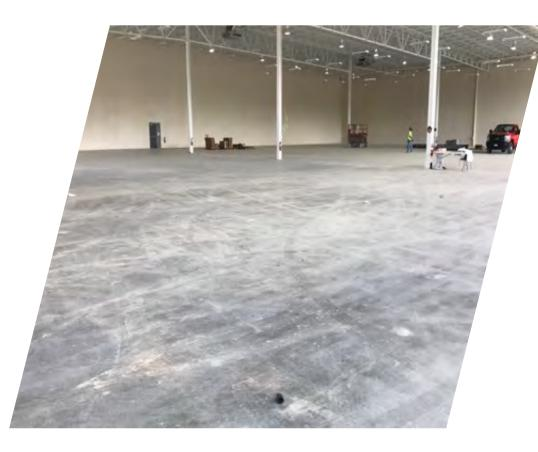
FRC slabs using low shrinkage concrete and extended joint spacing
