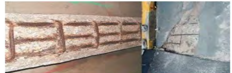
Corroded RC structures
