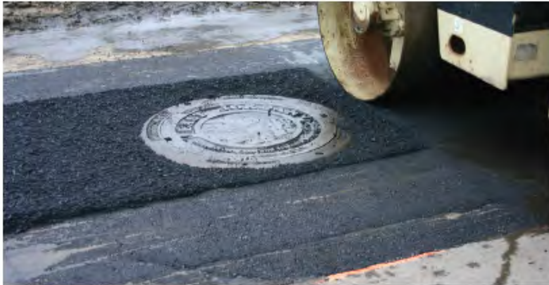
Step 6: Compacting
