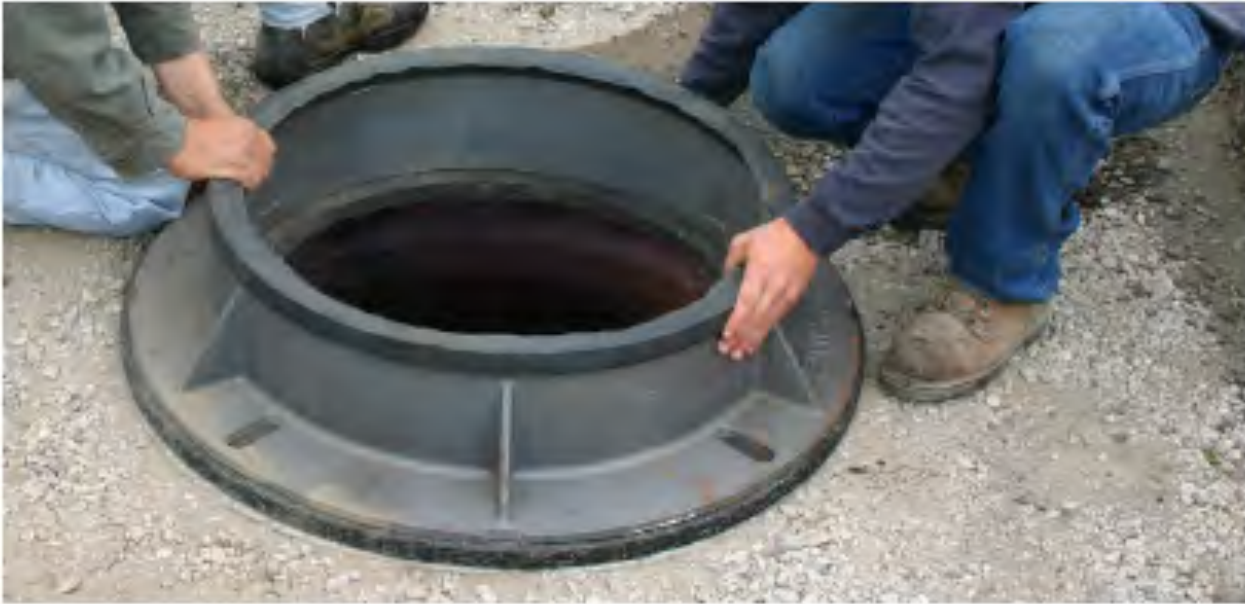
Step 1. Install Guide Frame
