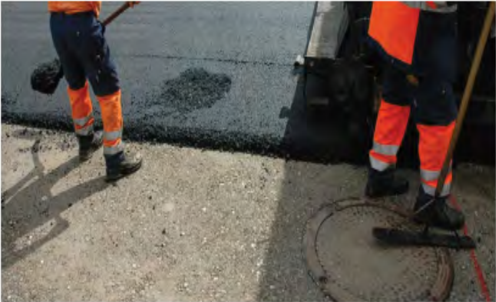
Step 4: Asphalt (top coarse)
