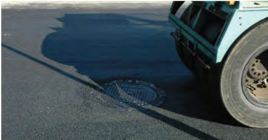
Step 7: Compacting
