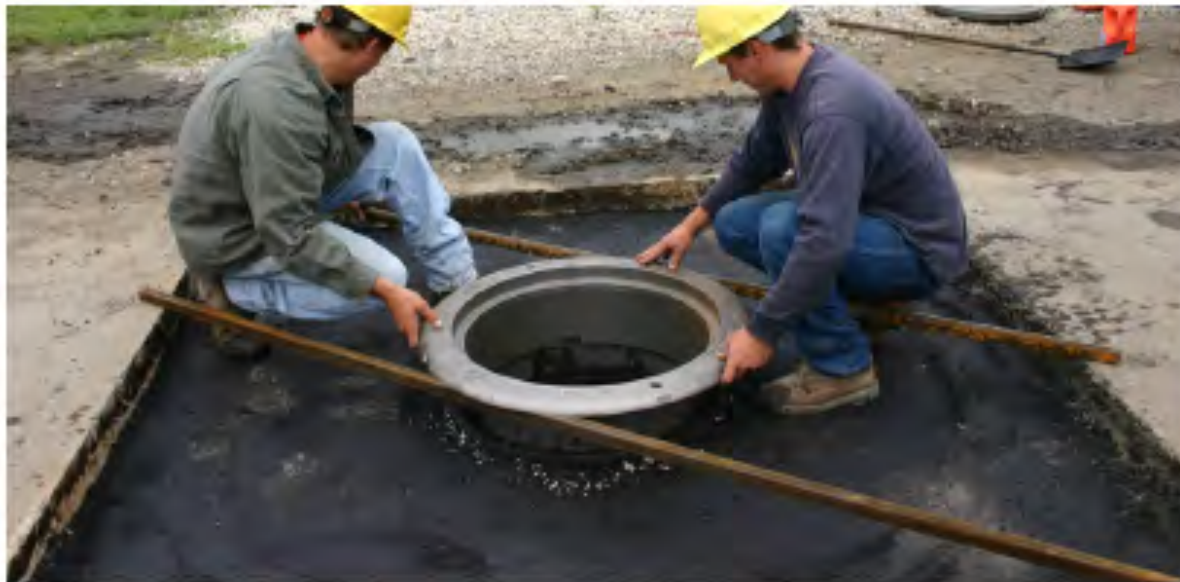
Step 4: Install Upper Frame
