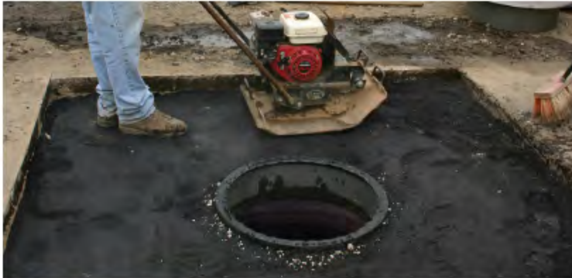
Step 3: Compact Backfill
