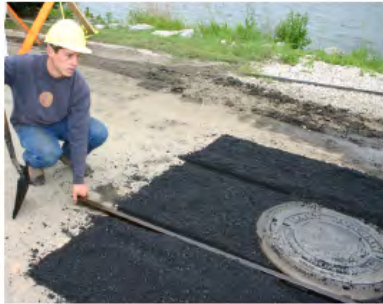
Step 5: Fill Remaining Asphalt
