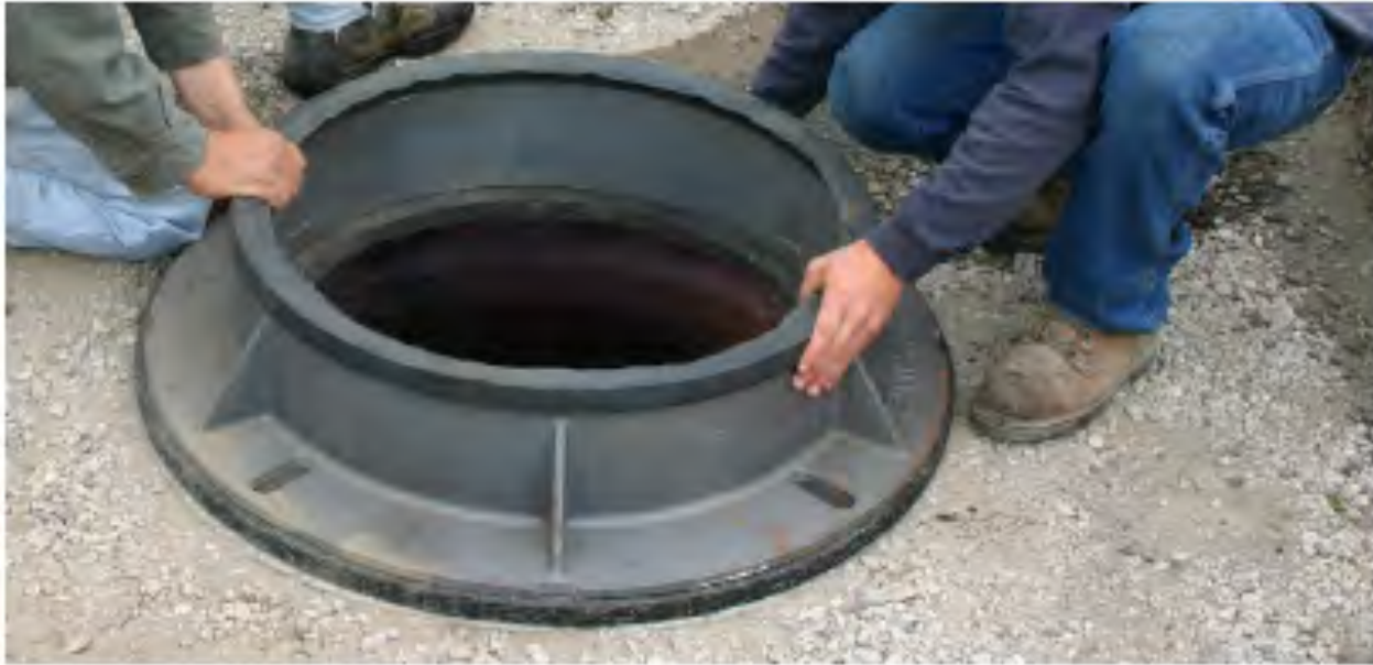
Step 1. Install Guide Frame
