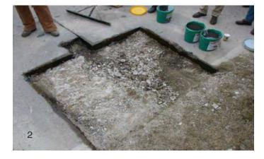
Place and Water the Cold Patch. 2 Degrees the night it was installed
