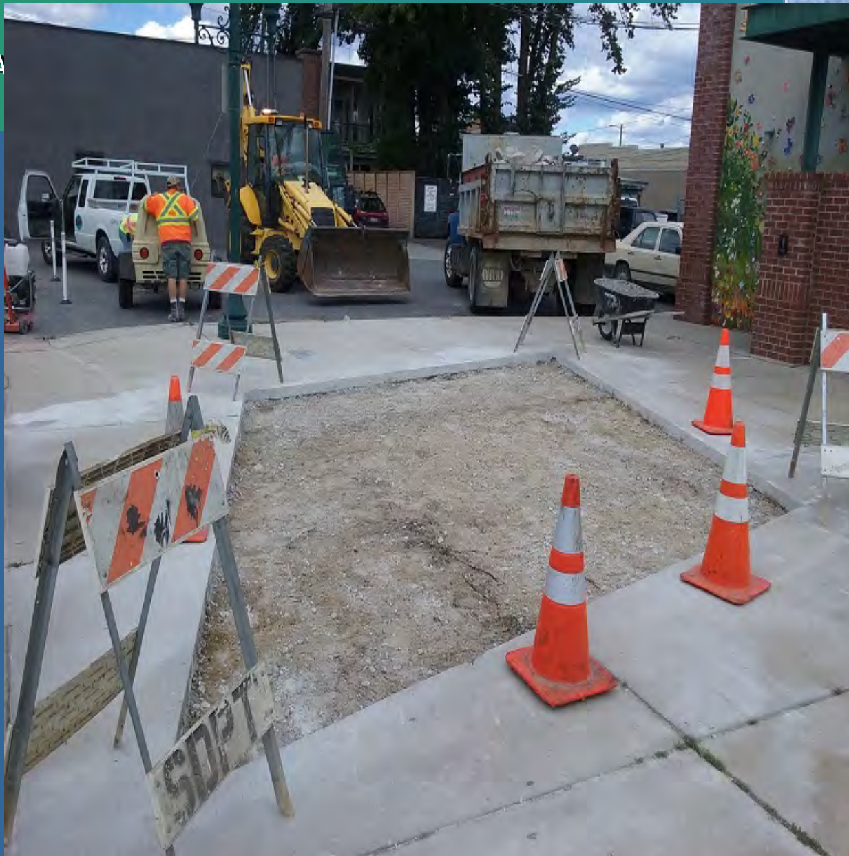
Existing concrete is cut
