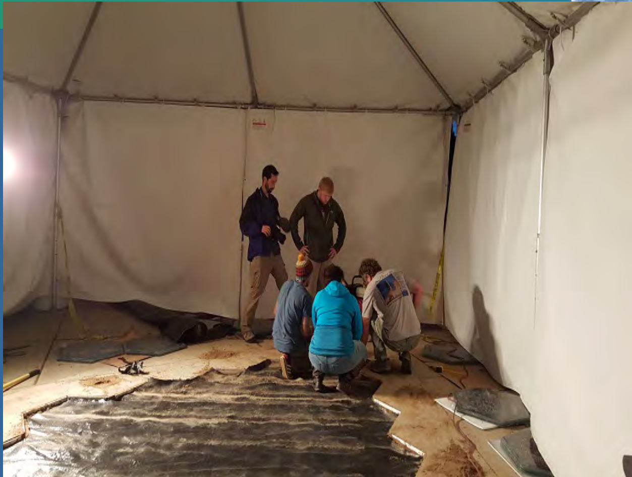
Installing Tyvar over the sand
