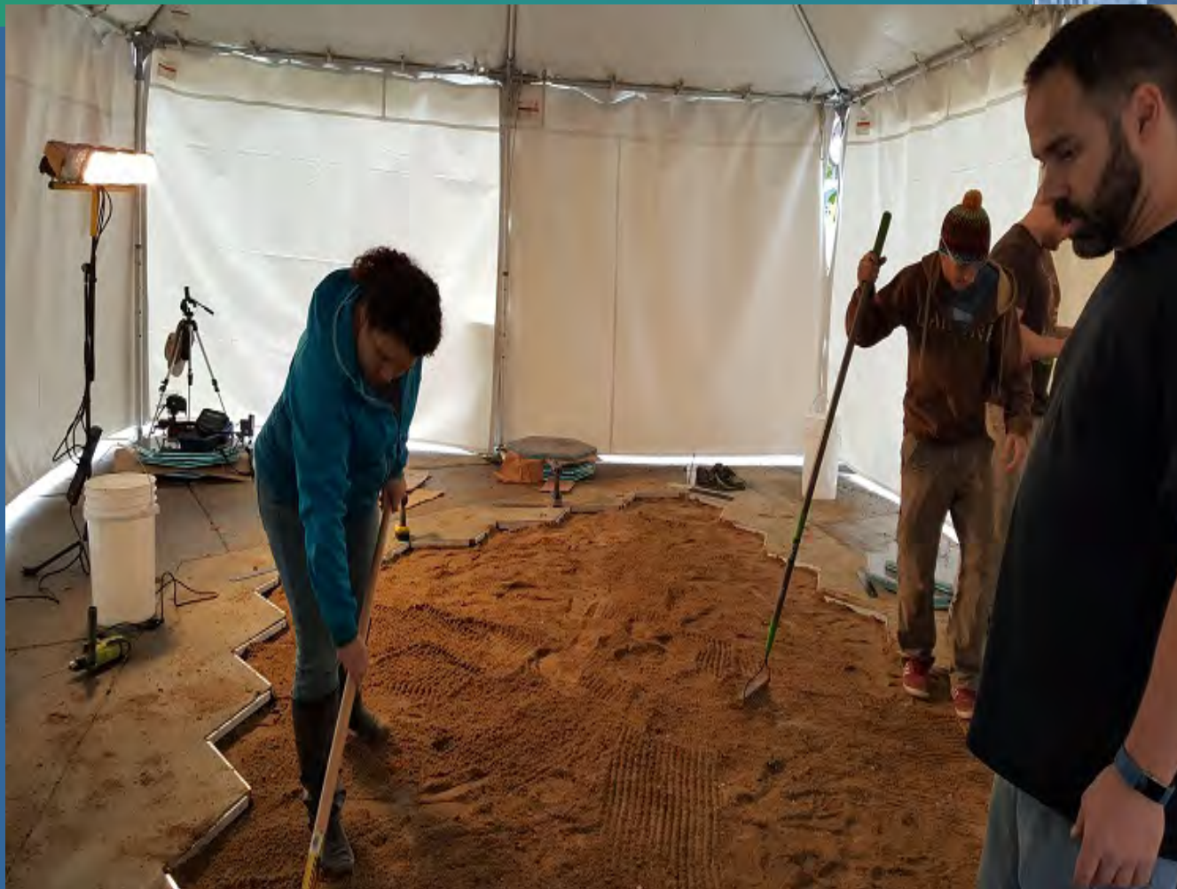
Leveling the sand base prior to compaction
