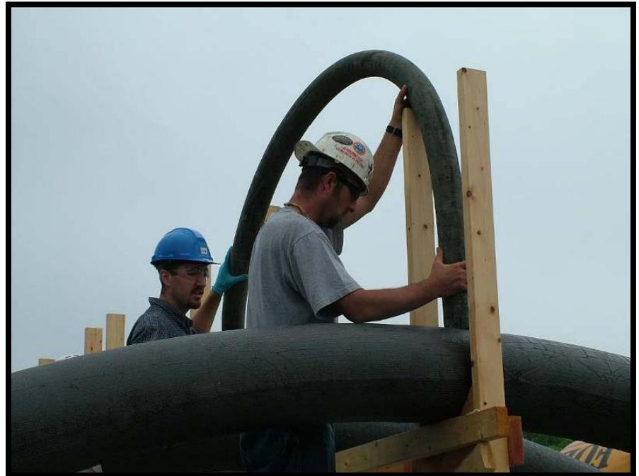
Concrete Filling of Stay-In-Place FRP Arch Forms
