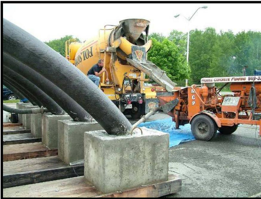
Filling Arches Using a Small Concrete Pump
