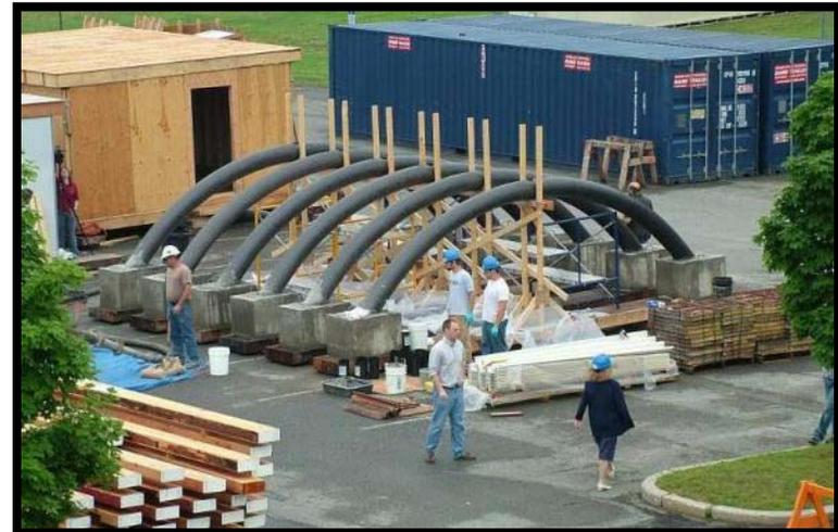
6 Arches Installed by 3 Laborers
