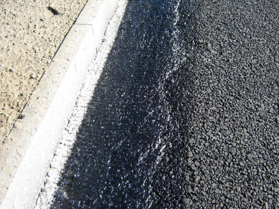
OGFC was placed at a 3.75 inch depth, and compacted to 3 inch depth.
