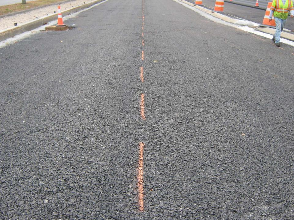
RS-1 emulsified tack coat used around all structures and curbline rather than PGAB 64-28
