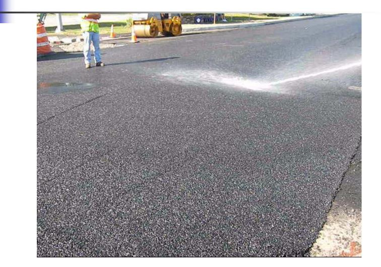
Mill and Overlay Sections 12.5mm w/ PGAB 76-28 SBS
